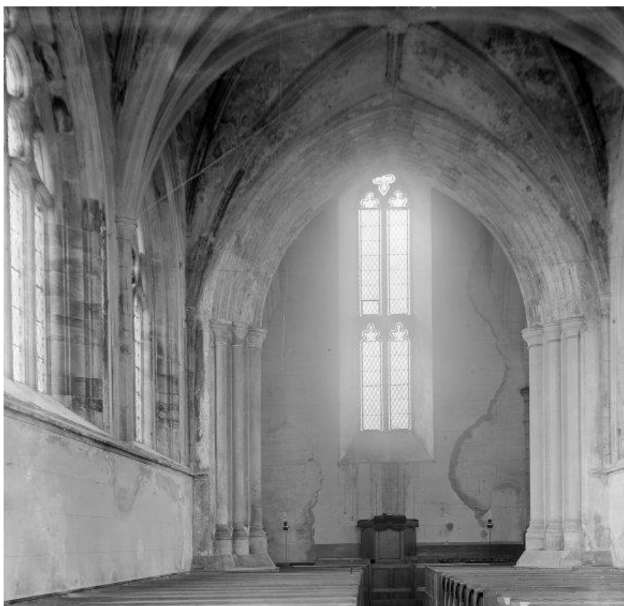
Fig. 16: Extent of damp and leaks, c. 1920 (c. HES/Canmore)
